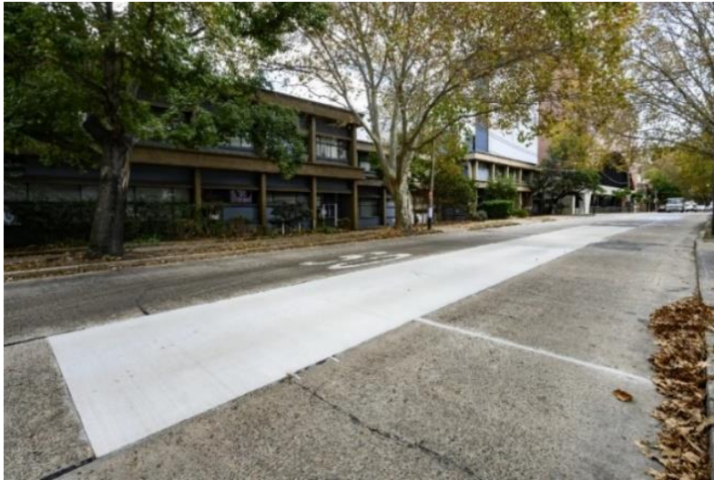
Figure 6.3 Road trial of Geopolymer with fly ash in Alexandria, Sydney (City of Sydney, 2019)
